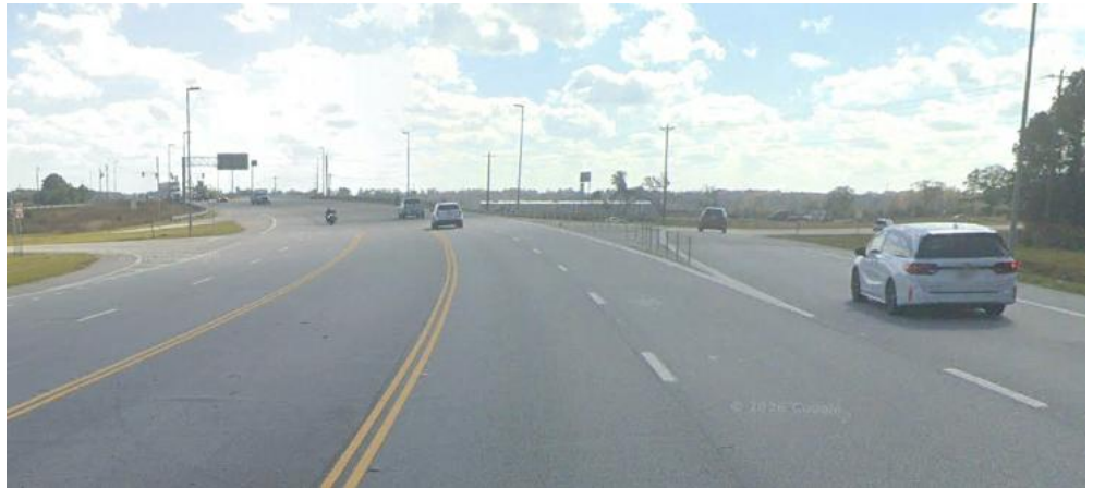
SC 327 (N. Williston Road) approaching the I-95 SB ramp. This area has had frequent crashes due to the lack of a traffic signal and drivers bypassing the loop ramp to turn onto the directional ramp. Bollards have been installed to prevent this action.
