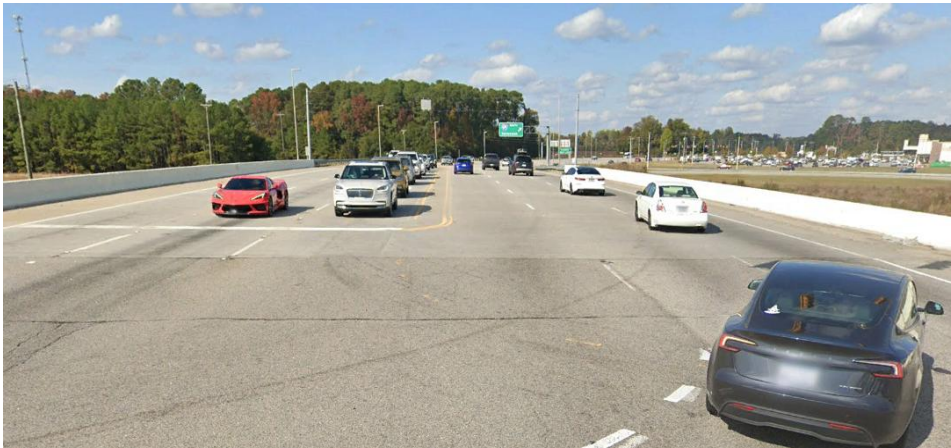
SC 327 (N. Williston Road) looking north showing the stacking of left-turning vehicles onto I-95 NB.
